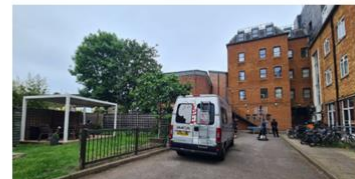
External courtyard / Service yard
