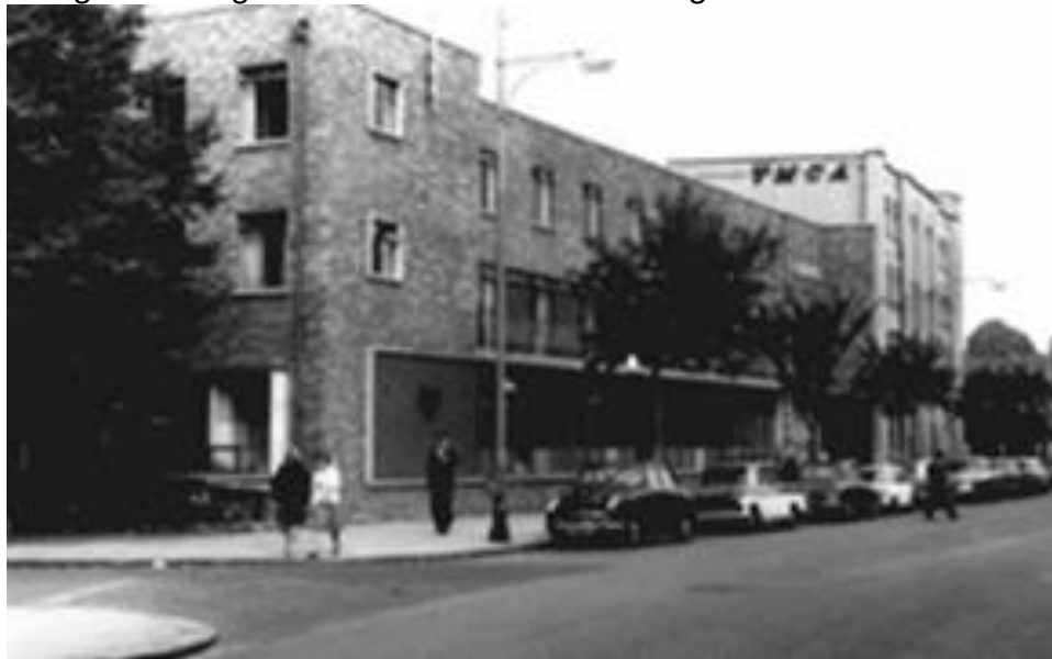
Figure 6 – Image showing the Sir Brett Cloutman Wing 1958
